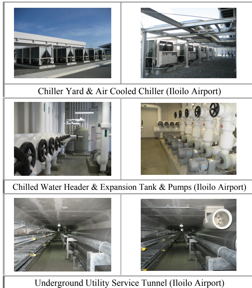
Figure 5.4-9 Chiller Yard & Chilled Water Pump Room
