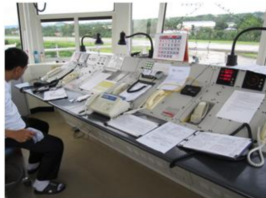
FSS Console inside of Tower
